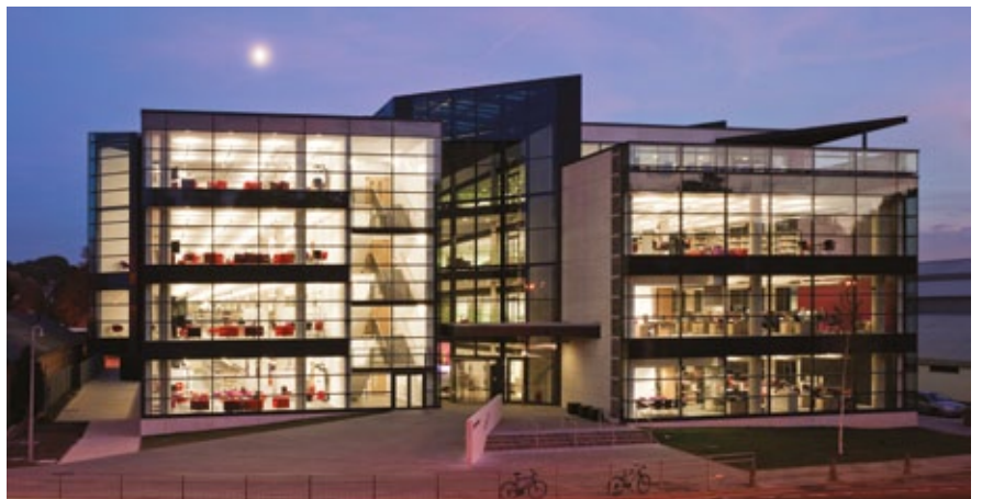
Canterbury Christ Church University Architect: ADP
